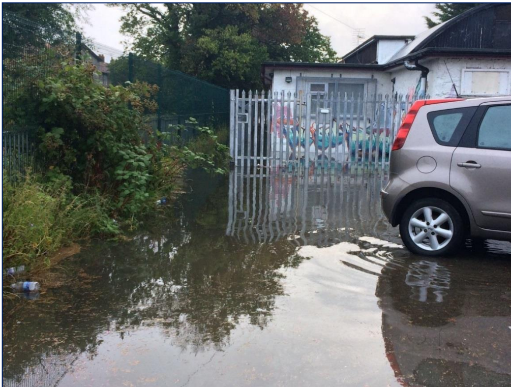
Figure 6: Flooding to Inferno Dance Studio. Front of the property
