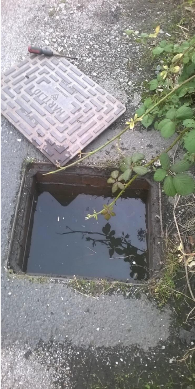
Figure 17: Inspection chamber directly upstream of outfall
