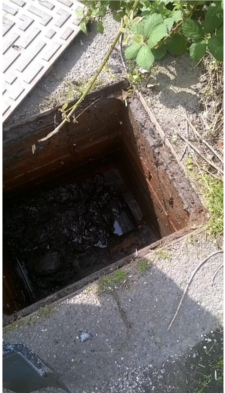
Figure 16: Chamber after the outfall de-silt
