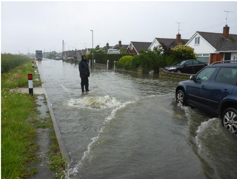
Figure 3 – Surcharging manhole cover on Ffordd Derwen
