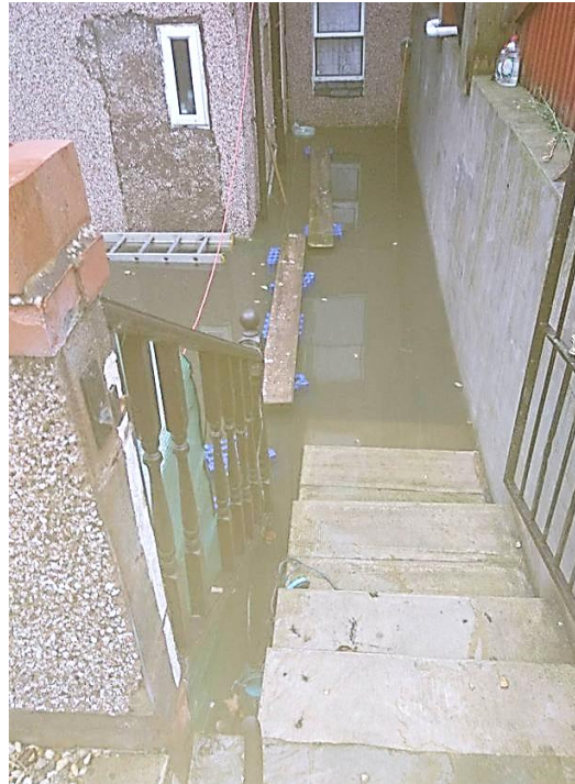
Figure 7 – Rear of Properties along Wellington Road suffered flooding due to a combination of surcharging combined sewer systems and surface water.
