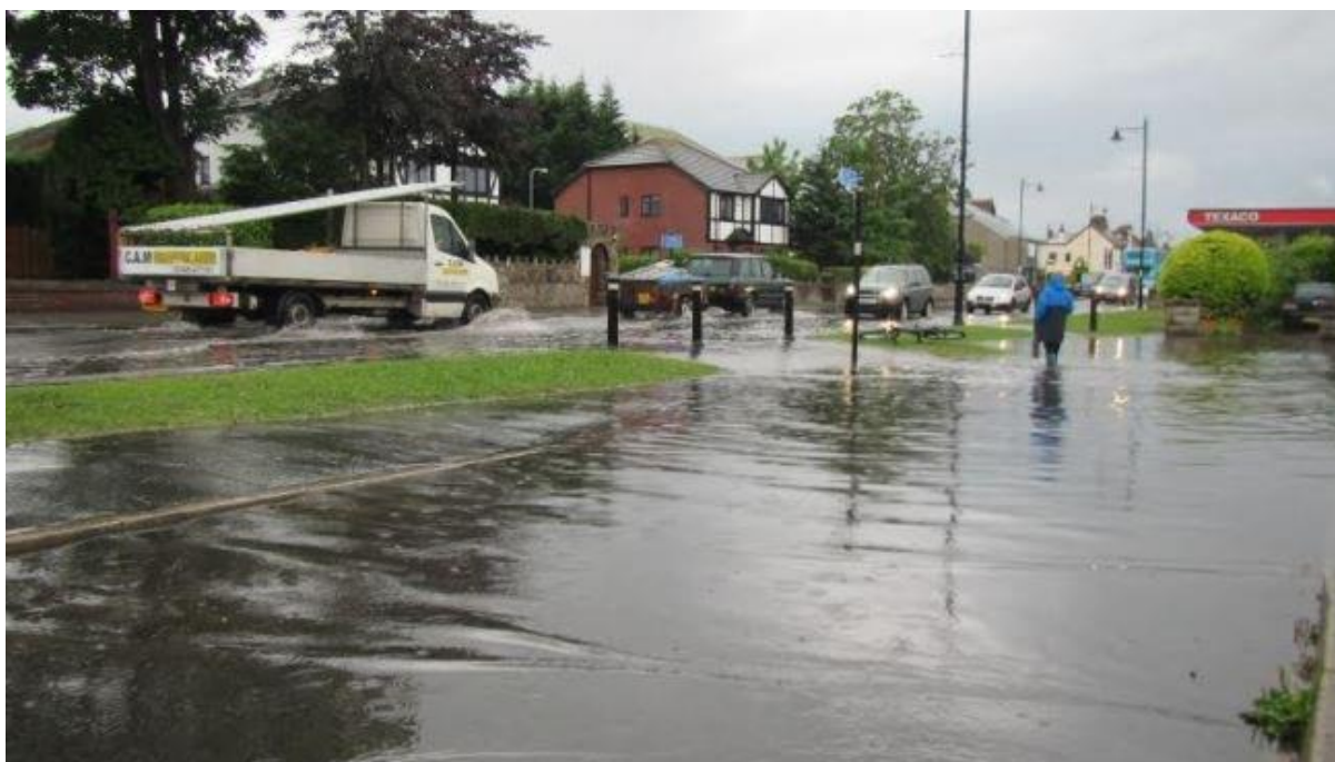
Figure 13 – Surface Water accumulating on Rhyl Road, Rhuddlan
