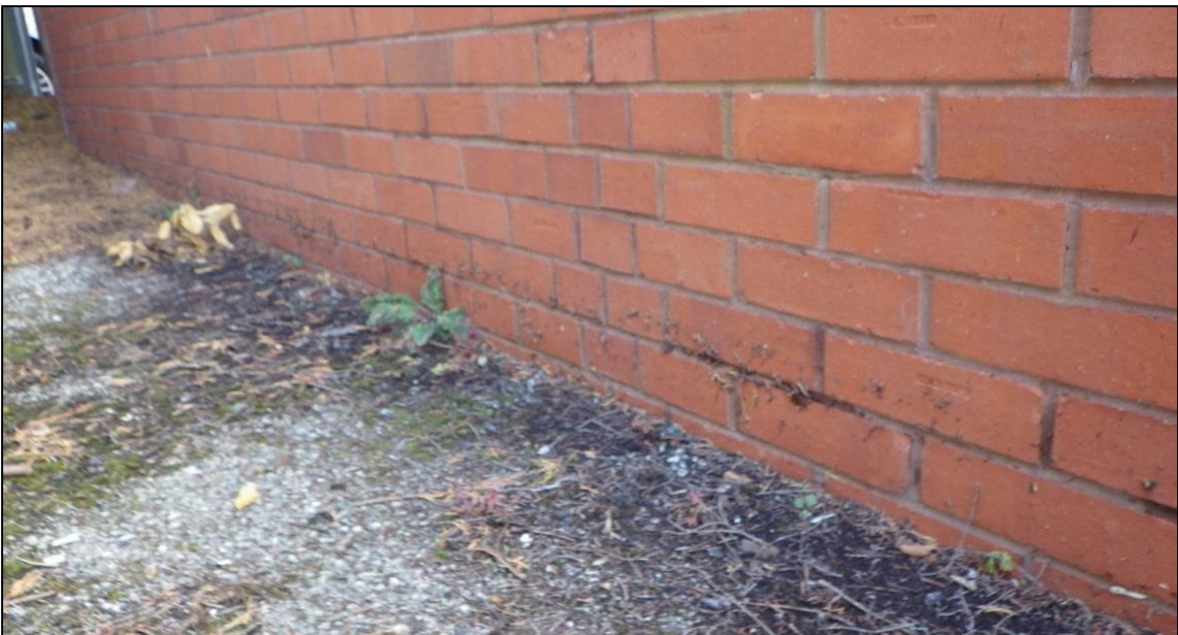
Figure 8: Wrack mark to Inferno Dance Studio rear yard wall.
