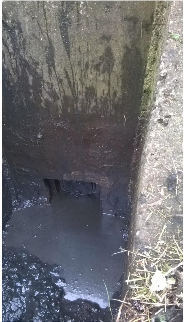
Figure 18: Post de-silt with metal flap valve visible
