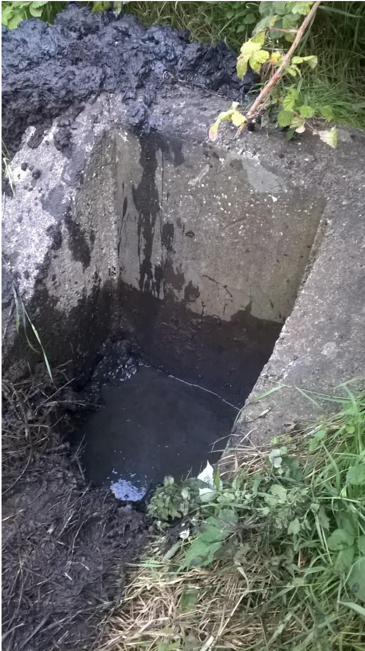
Figure 19: Outfall after minor silt removal
